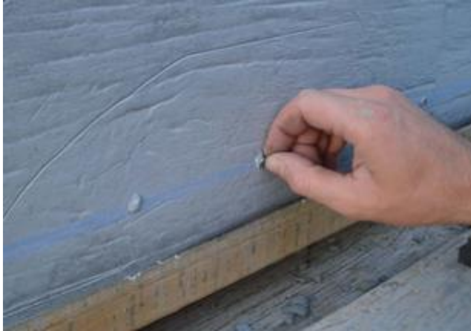
Figure 2-2. Placement of DEMEC points (Photo by author).
